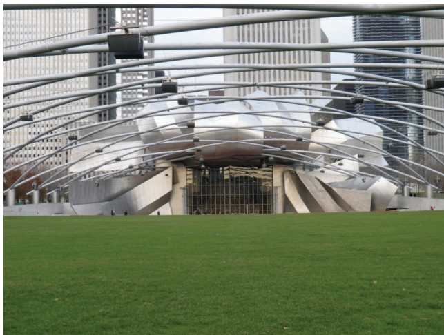
Figure 5. Millenium Park green roof Chicago ( source author )
