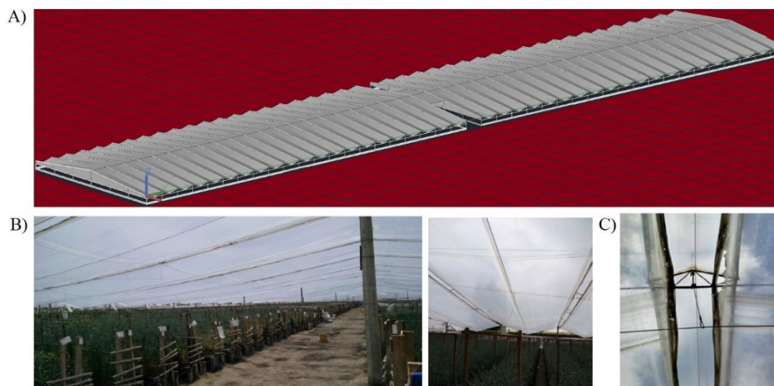
Figure 1. A) General scheme of the space greenhouse, B) Details of the interior of the greenhouse and C) Ventilation area
