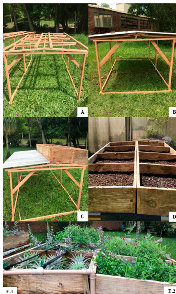
Fig. 2. Illustrations of the prototype built to receive the next layers of the green roof system are shown and after installation. In (A), the base of the structure is depicted; in (B), the base is shown after receiving the fiber cement tile; in (C), the prototype with a box is illustrated; in (D), the prototype is depicted already installed and filled with pine bark substrate; in (E), one of the blocks with developed plants is shown. Subsequently, (E.1) shows the drip irrigation system, and (E.2) shows the block without an irrigation system.
